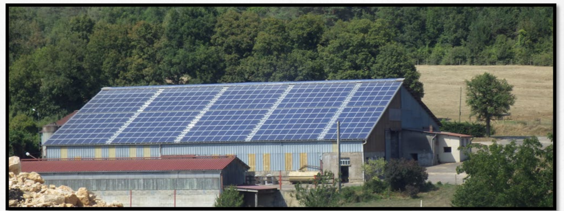
Installation photovoltaïque en revente _ GAEC Tonnot
